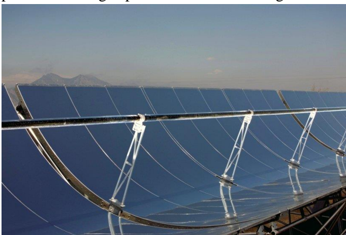
Fig Parabolic Trough Collector
